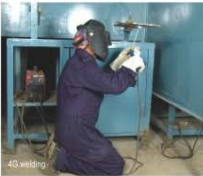
Stainless Steel Welding
